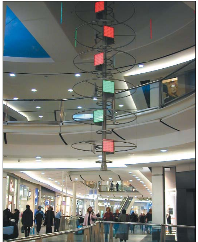
Fig. 1. A 14 m suspended LED tile fixture in the Centrale shopping mall in Croydon, UK, provides an exciting decorative effect.
