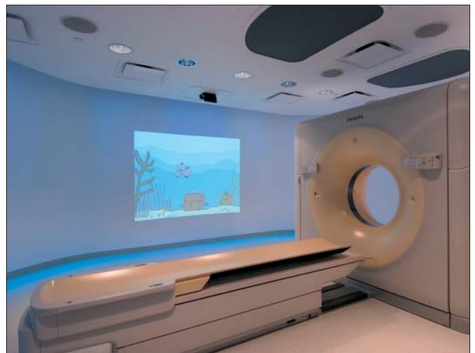
LED cove lighting around the curved walls of the radiology suite at this children’s hospital provides a changeable ambiance that can result in a more patient-friendly environment and improved care.
