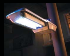
Solar powered streetlight
