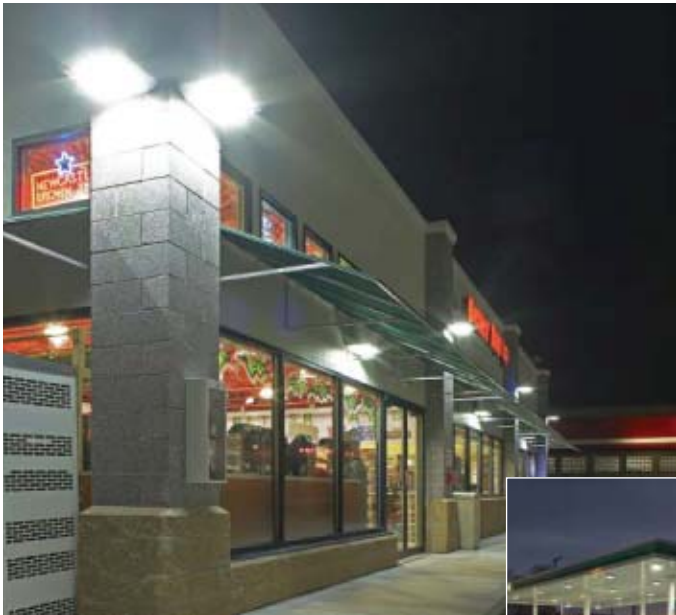
Wall-mounted LED fixtures (four LED bars each) around the building at the Better Day BP.
