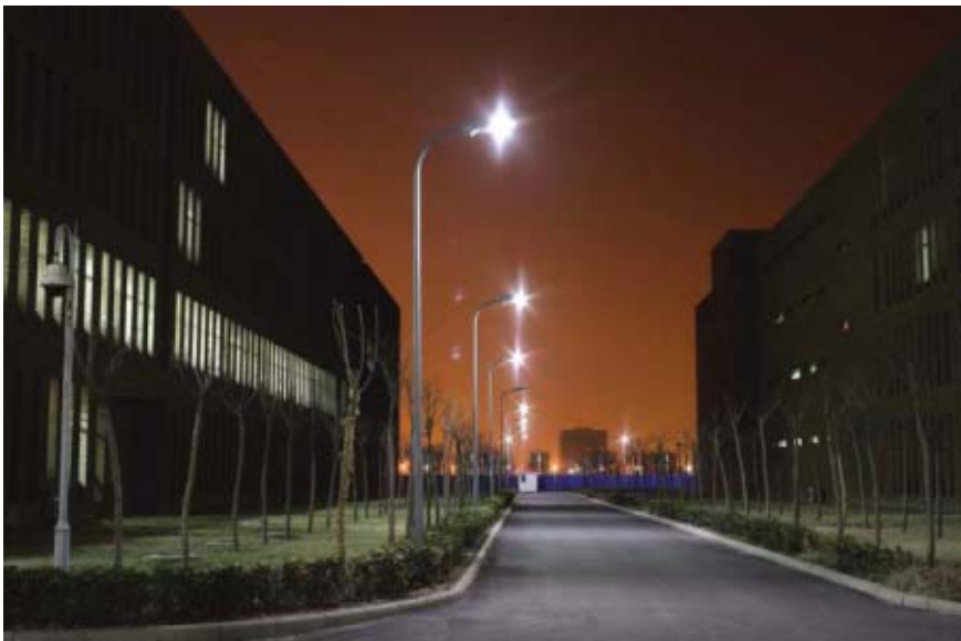
LED streetlights installed at the Tianjin Polytechnic University campus
