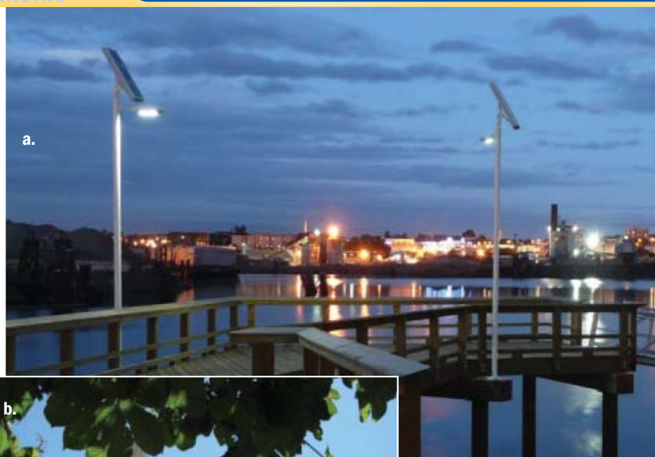
FIG. 5. (a) Solar-powered LED area lights illuminate harbour ferry dock in Victoria, British Columbia. (b) Installation of solar-LED light fixtures.
