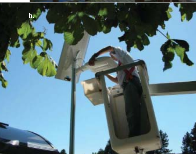
FIG. 5. (a) Solar-powered LED area lights illuminate harbour ferry dock in Victoria, British Columbia. (b) Installation of solar-LED light fixtures.
