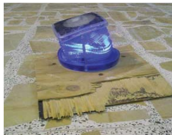
FIG. 3. A durable solar-LED taxiway light continues to operate even after being run over by an airfield service truck.
