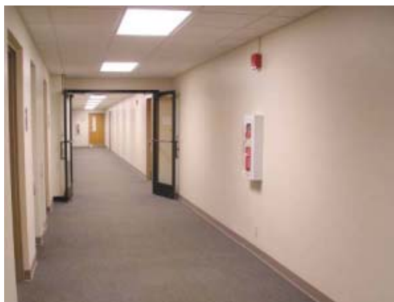
ilumisys installation of first-generation MK1 tubes in the Escanaba, Michigan, State Office Building.
