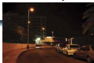
HPS Street Light
