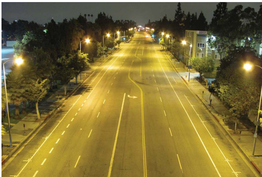
FIG. 1. HPS street lights on Hoover Street in Los Angeles near the University of Southern California campus leaves dark areas along the major street.
