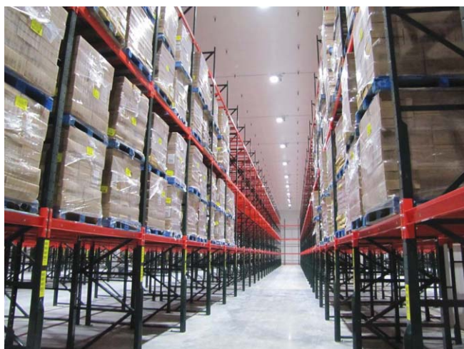
Metal-halide lamps (top) and solid-state lighting (bottom) in Americold cold-storage warehouses.
