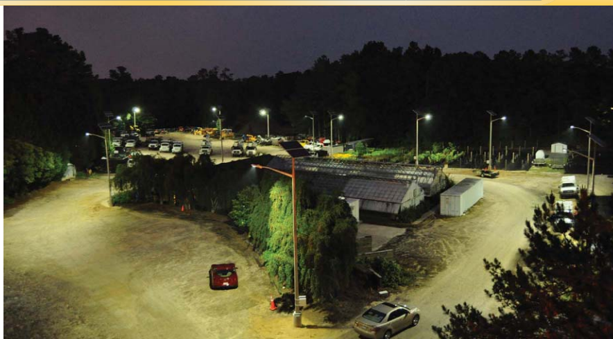
Raleigh combined solar cells and LED lighting at a remote operations center.
