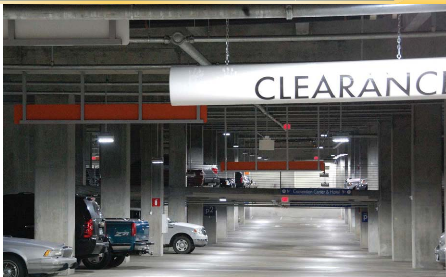
LED lighting in the Raleigh convention-center parking structure.
