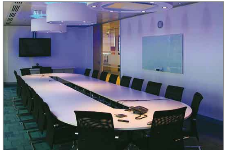
Figure 4: Meeting room entirely lit with solid-state fixtures
