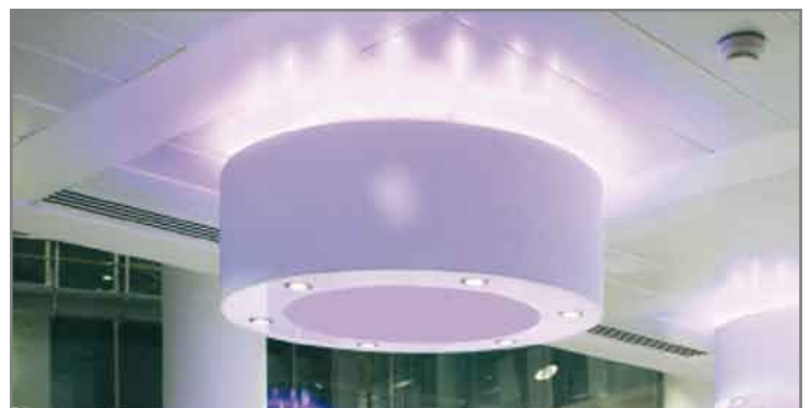
Figure 5: The fixture is equipped with warm white LED light engines for task lighting and blue LEDs for ceiling accent lighting
