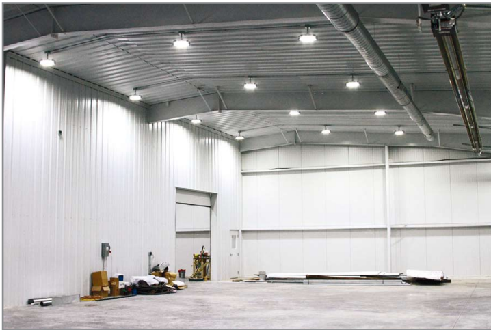
Figure 1: Frontline's new processing facility with LED High Bays from 7 metre high ceiling.
