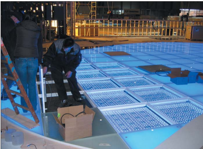
Fig. 4. The installation of LED floor panels at the Lexus booth.
